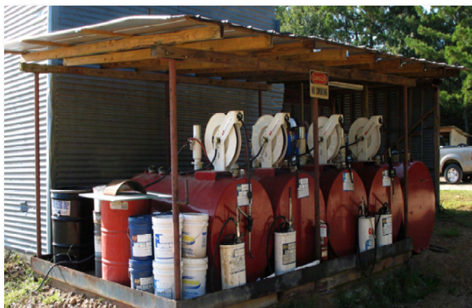
Oil Storage – TXI Double wall tanks
