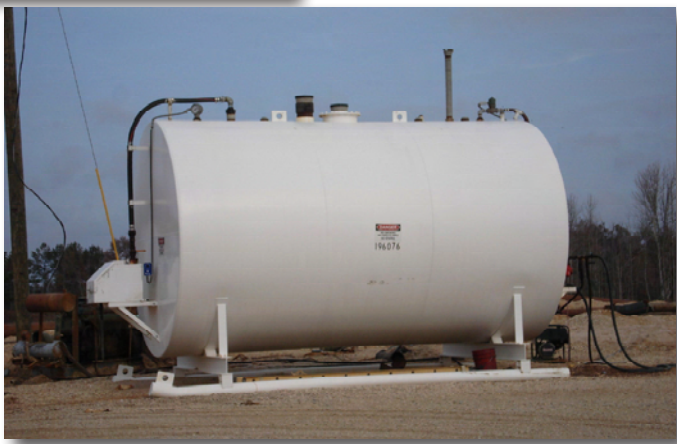
Oil Storage – Double-wall Diesel AST - MMM
