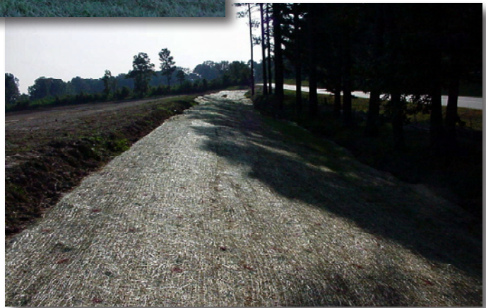
Erosion control blanket use – TXI vegetative control
