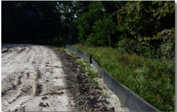
Silt fence utilization – TXI structural control
