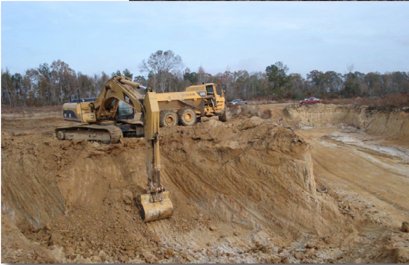
Overburden Stripping Activities - MMM
