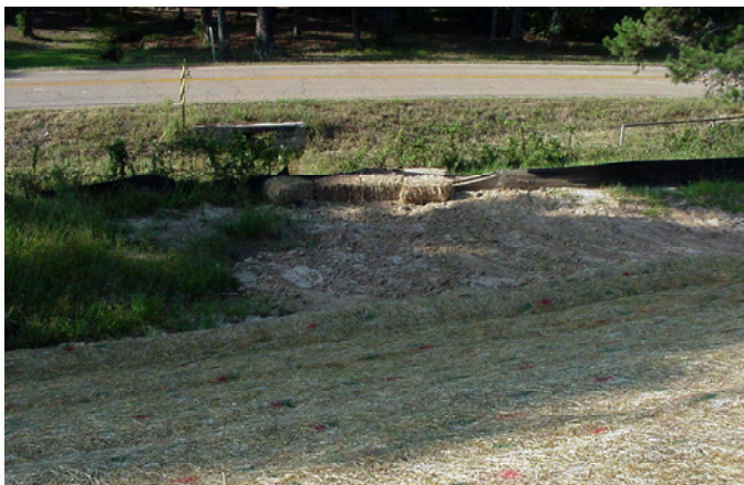
Silt fence and straw bale usage - TXI straw bale, silt fence and matting BMPs
